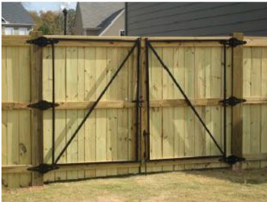
Acceptable gate – interior hinges, fully supported, No large gap between gate and ground.
