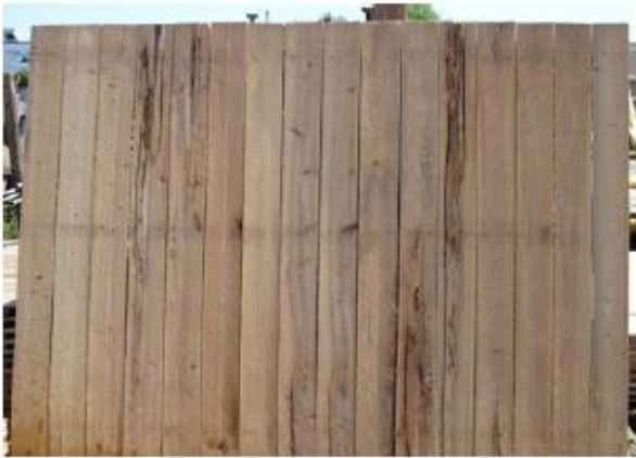
Unacceptable; no finished on top
