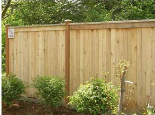
Style 1: Acceptable; fencing capped on top
